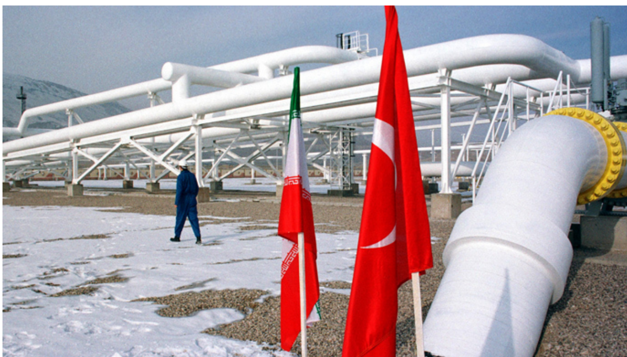
A worker walks past the pumping station on the border between Iran and Turkey (Reuters)
