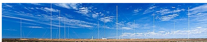
VLF antennas at Harold E. Holt Naval Communications Station, North West Cape
