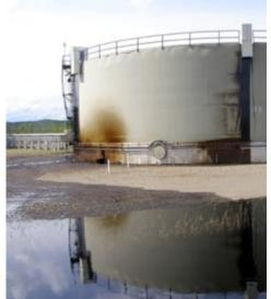
Tank 190 is surrounded by a containment area that has an impermeable liner. (Photo: Alyeska Pipeline Service Company)
