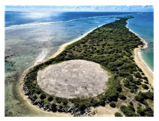
"Seawater is penetrating the underside of the dome, because when they threw all this material into the old bomb crater, they didn't line it with anything. They were supposed to line it with concrete, but that never happened because of cost considerations. So, as the sea level has risen, the groundwater level has risen and therefore you have groundwater penetrating inside the dome, because a lot of this atoll is obviously sand (and) coral. It's permeable material."
