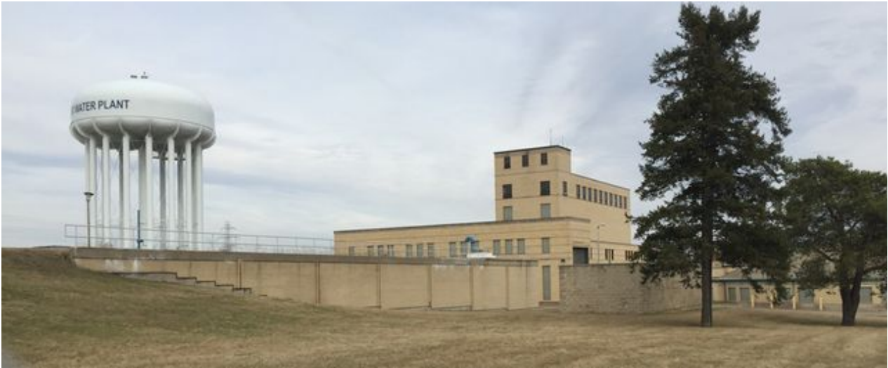
Image: The Flint water treatment plant
