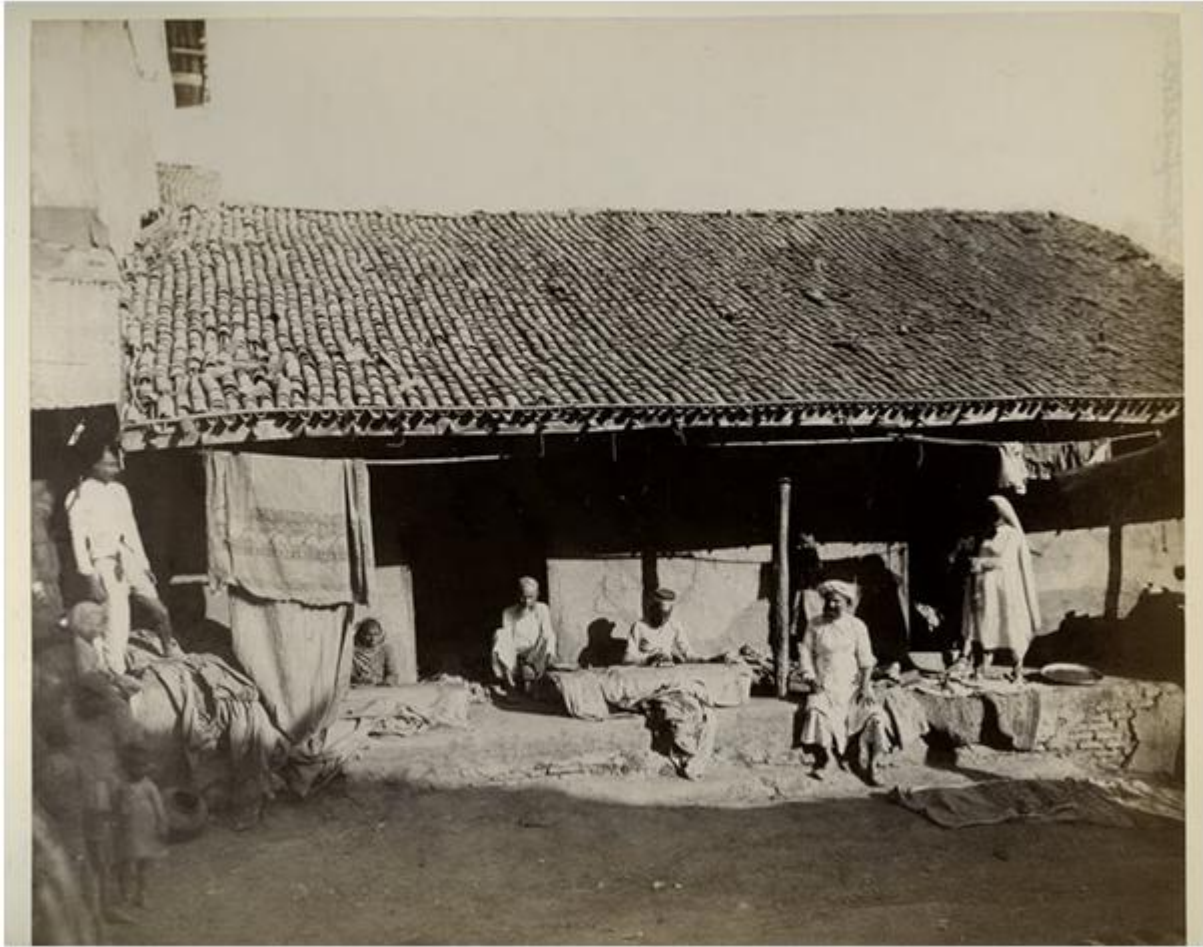
Image 1: Farmer's hut, 1880; these huts were better suited to the harsh Indian summer and the equally harsh winters. The clay tile roof not only drained rainwater, it insulated the home from heat and cold. These hollow clay tiles with air pockets insulate the home from the top. The clay walls keep the homes cool.
